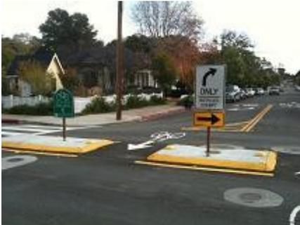
**Streets with traffic calming features and speed limits of 20 mph or less:** Streets with speed limits of 20 mph or less that use physical and visual cues to encourage motorists to drive more slowly. The design of these streets is self-enforcing; the design of the roadway results in slower motorist speeds and comfortable bicycle riding without relying on compliance with traffic control devices such as signals and signs.
